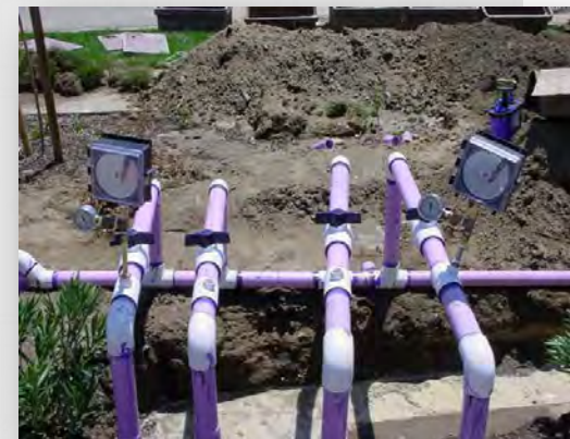
Shut-down test on irrigation system
