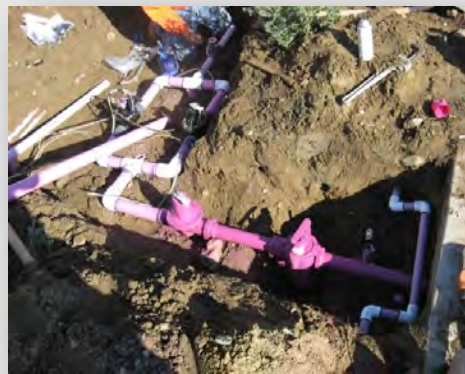
Building the irrigation system & inspecting before covered
